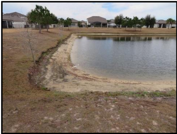
Figure 3 - Pond 28 Shoreline Erosion
